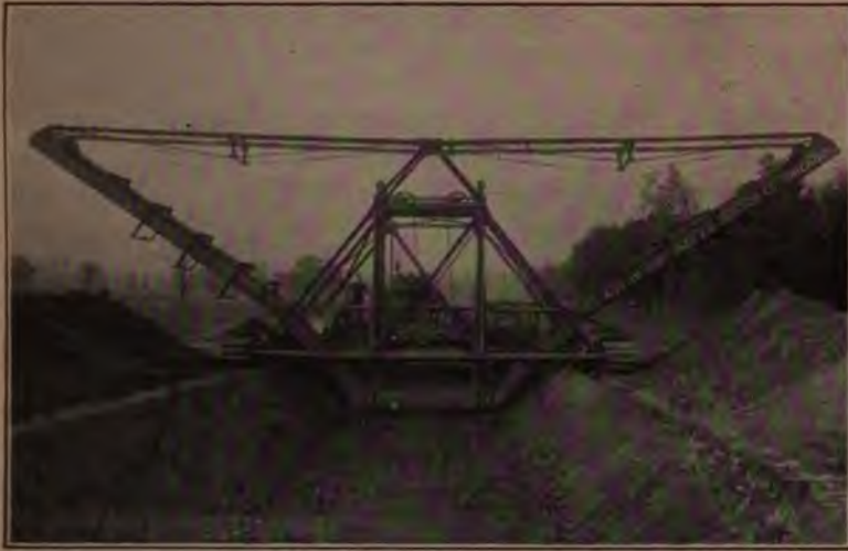
Austin Templet Excavator with Wide Bottom Frame. Figure 58.
